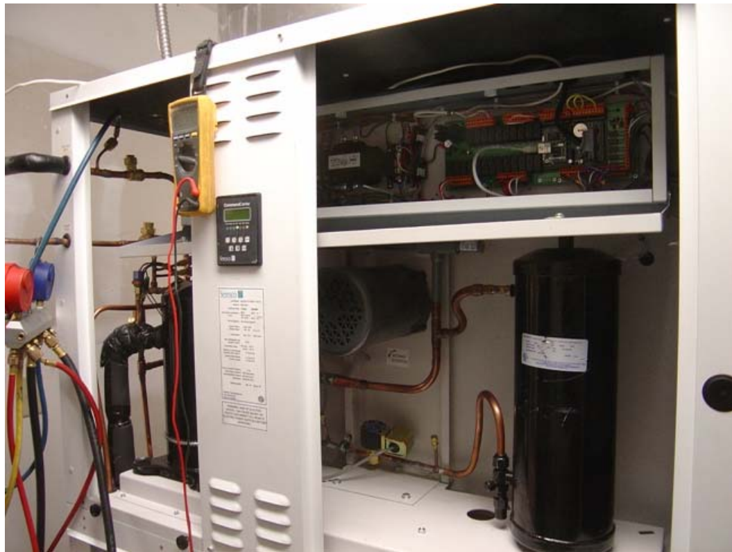
SERESCO™ NE SERIES POOL DEHUMIDIFIER'S INTERNAL CONSTRUCTION
