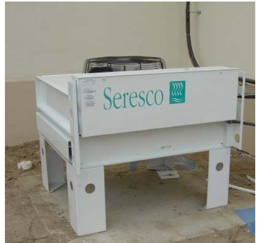
RIGID CONSTRUCTION & STRUCTURE OF THE OUTDOOR AIR COOLED CONDENSING UNIT
